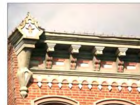
Above: Example of restored metal cornice
