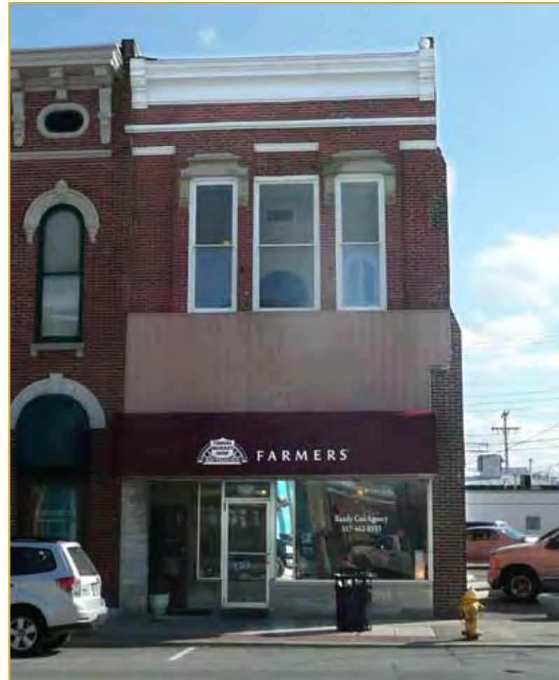
Above: Existing facade
