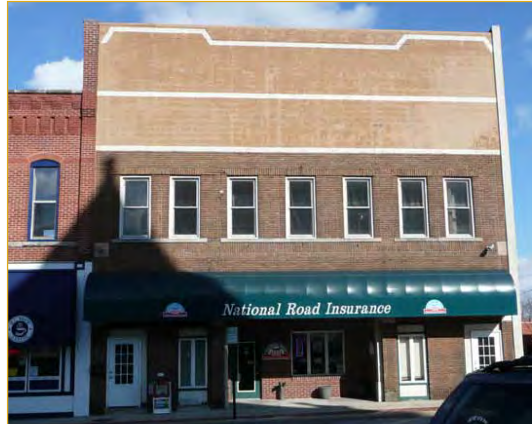
Above: Existing facade
