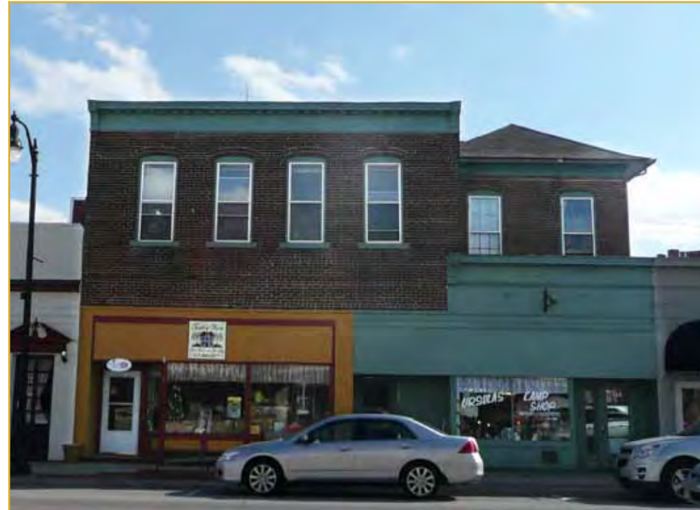
Above: Existing facade
