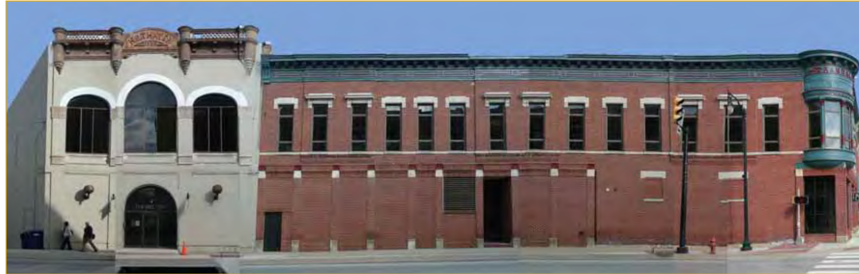
Above: Existing facade
