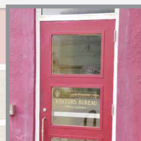
8 Main St: Visitor's Center- Adjacent theater looks great, but the stairs might be a problem for some. Also, nothing posted about operating hours or public rest rooms.
