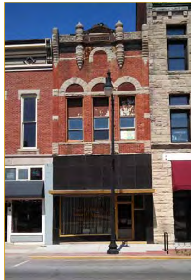
Above: Existing facade
