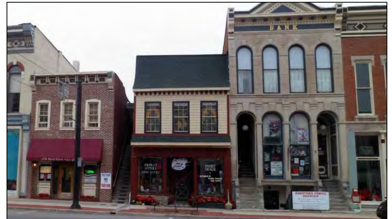
Above: Compact, attractive storefronts promote window shopping.
