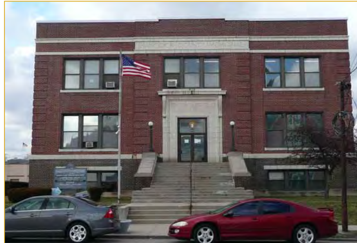
Above: Existing facade
