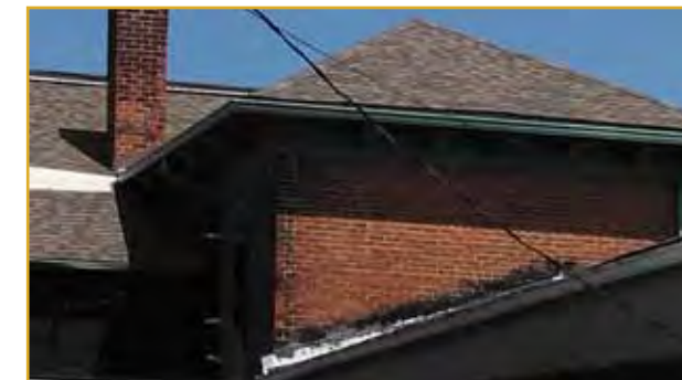
Above: Rear roof detail including residential building
