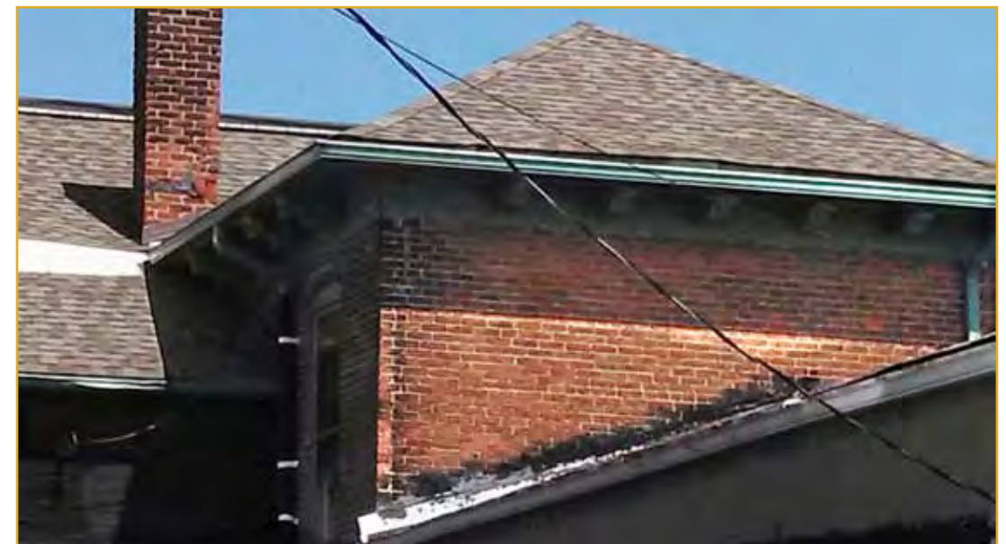
Below: Gutters and roof detail
