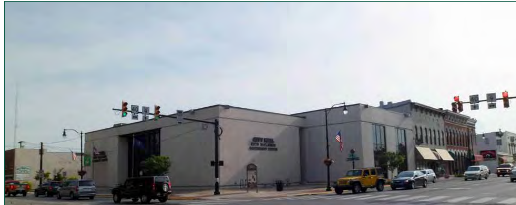
Above: City Hall at U.S. 40 and S.R. 9; June 2013
