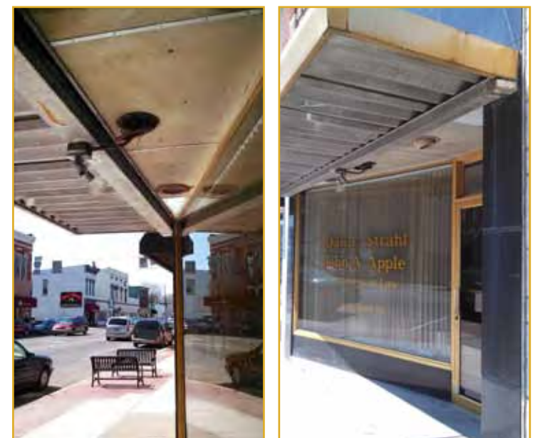
Above: L.A. Davis metal awning
