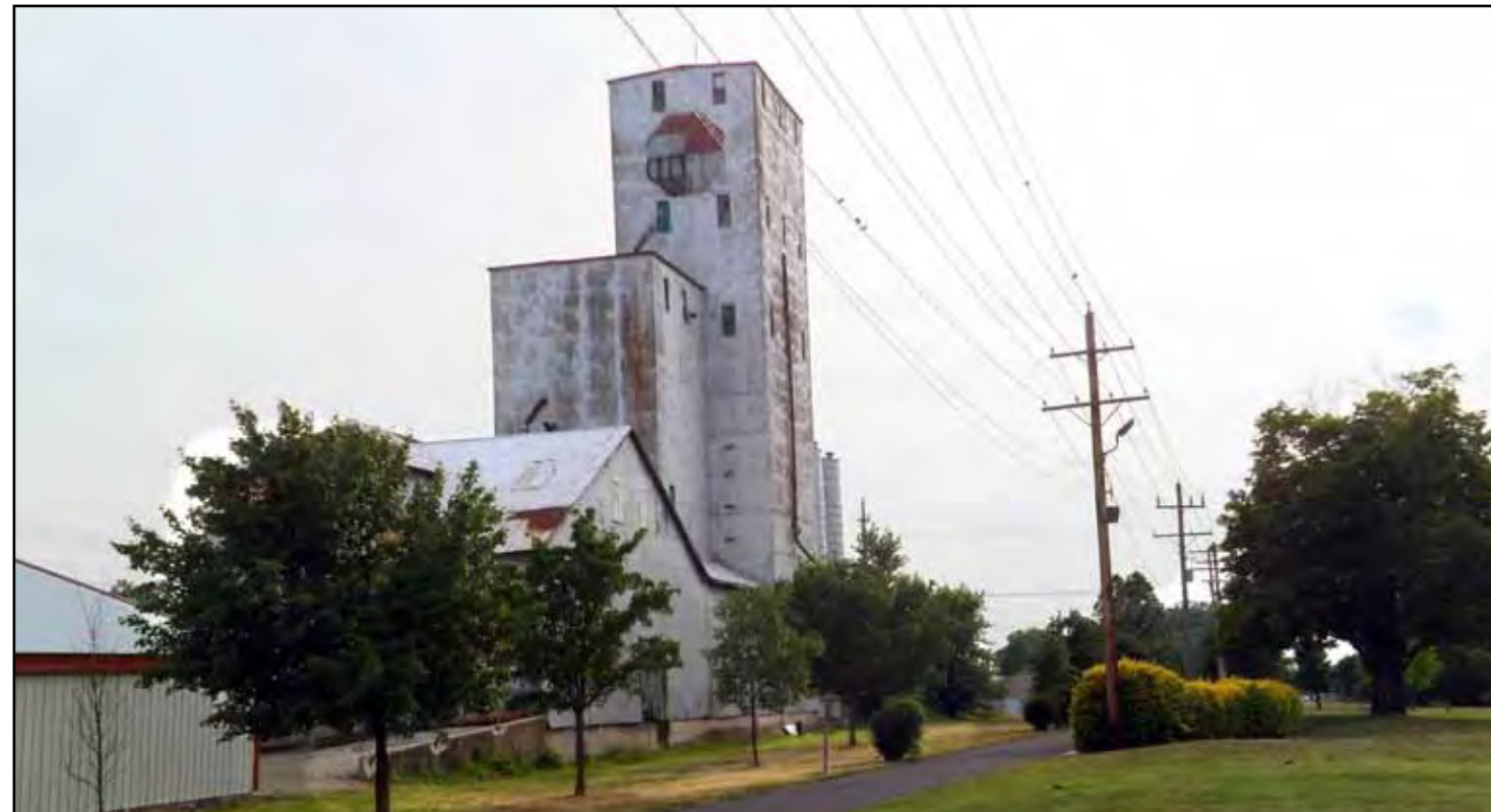
Below: Pennsy Trail West of Pennsylvania Street
