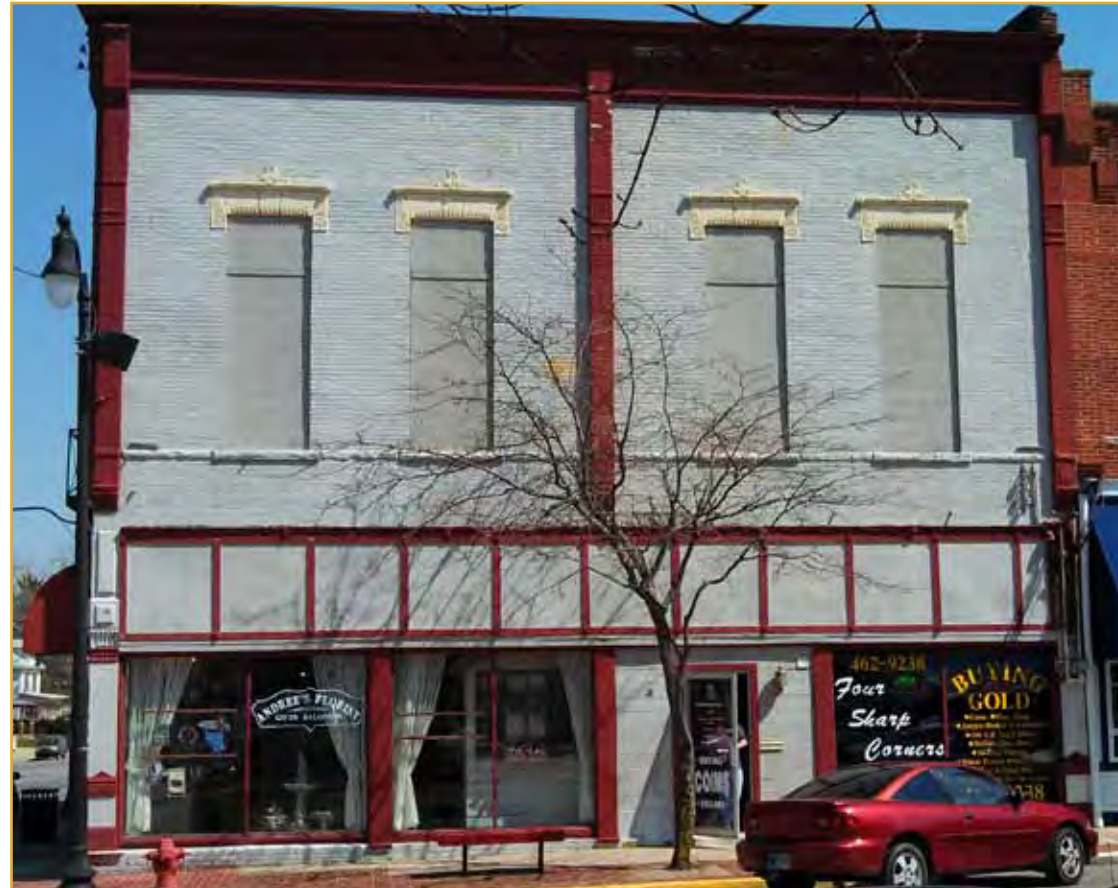
Above: Existing facade
