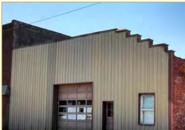
Above: Parapet wall example
