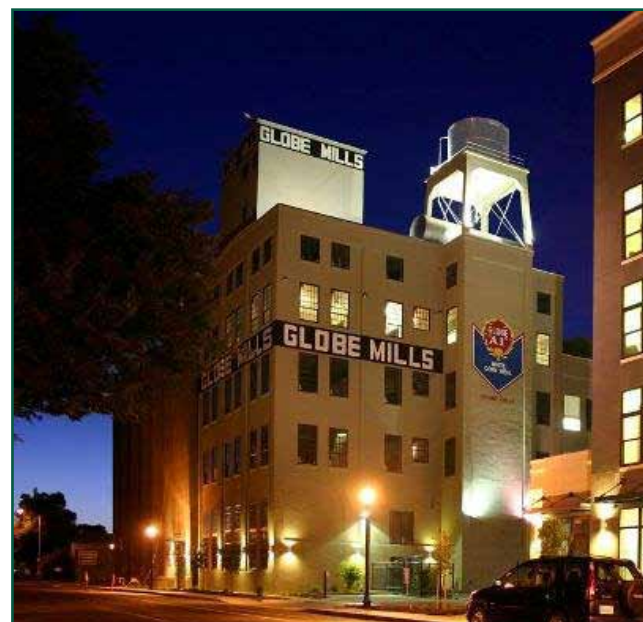
Below: Globe Mills Grain Elevator, Adaptive Reuse, Sacramento, California
