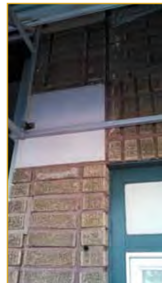
Above: Detail of brick and vinyl awning
