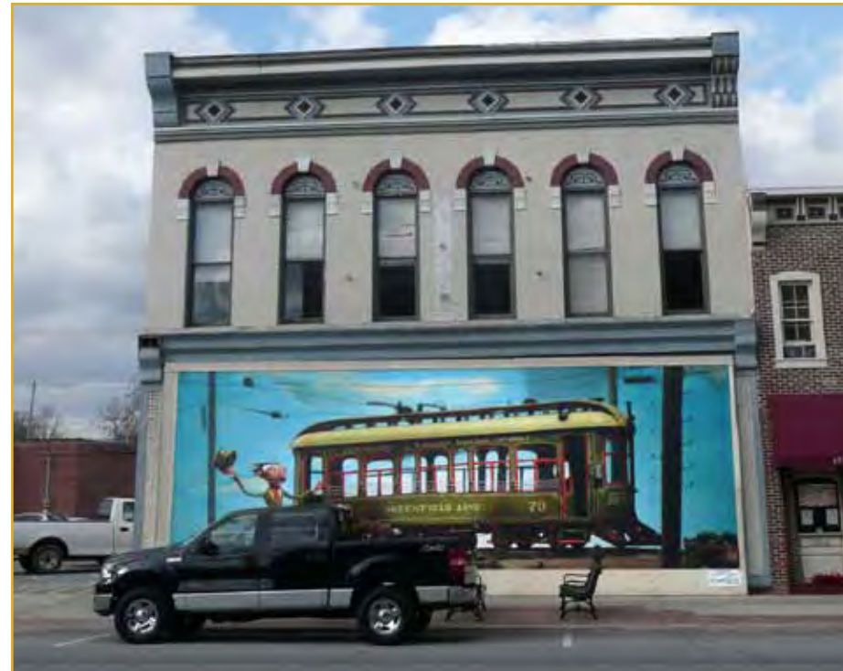
Above: Existing facade
